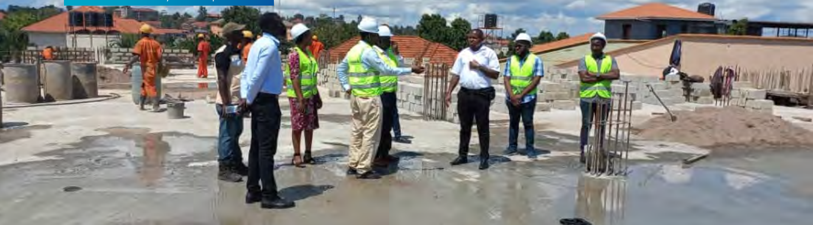
Council members inspecting progress of works Pharmacy House phase II
